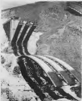
Chiseled out of the side of one of the Andean foothills, Bridge No. 1 is the largest concrete bridge in America and the fifth longest in the world. It is one of the highway's three bridges.
